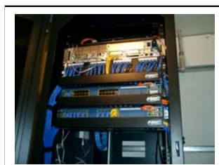
New EEC Network Installation
