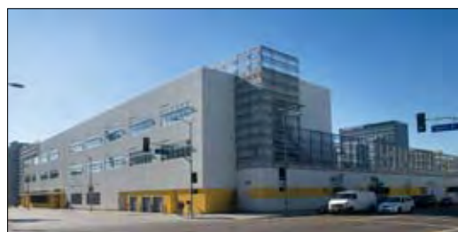
Central LA Area New MS #3 - Completed
