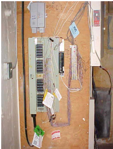
Existing Telephone Wiring Termination Installation
