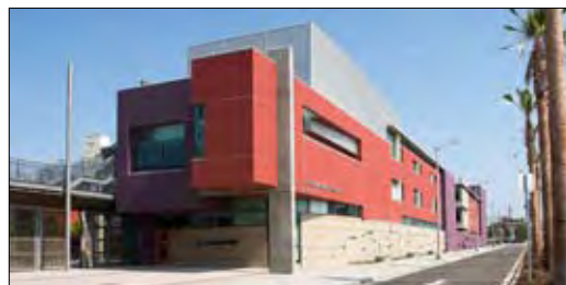
East Valley Area New MS #1 - Completed
